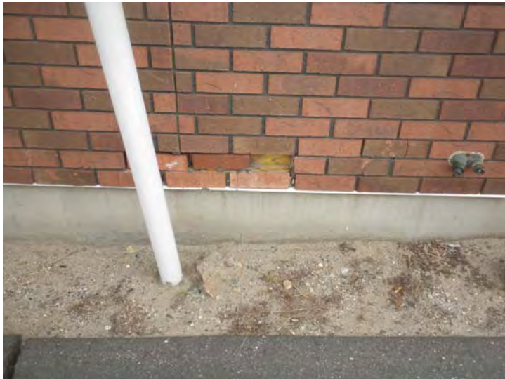
Example of damage to the EFIS siding
