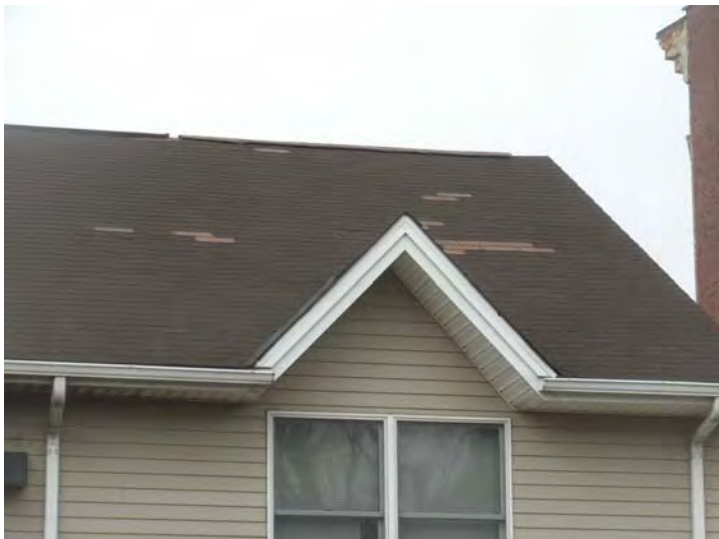
View of the roof area with replacement sections
