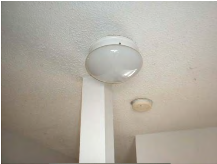
Typical light fixture and living area smoke detector
