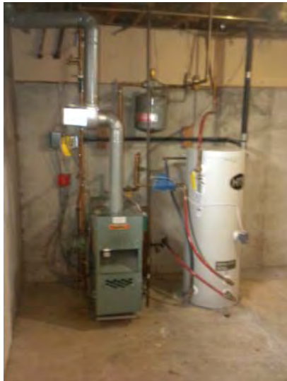
Boiler and in-direct domestic hot water tank (located in a basement)
