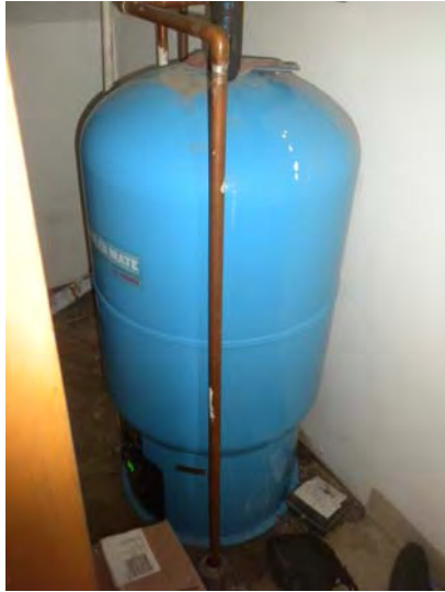
Original in-direct domestic hot water storage tank
